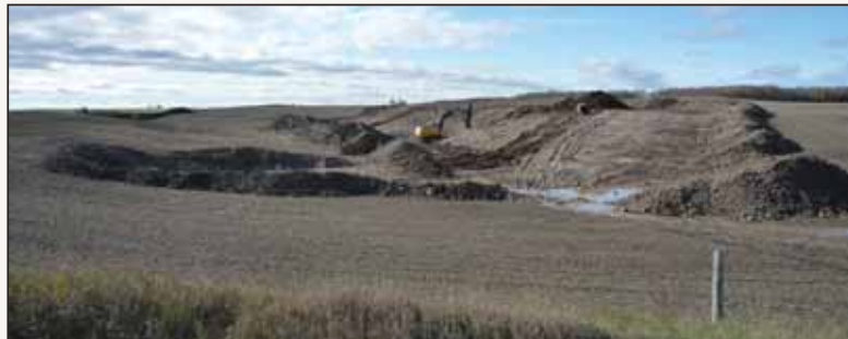
Berm construction underway at the Eadie farm. Berms slow down stormwater drainage, reduce erosion and retain farm topsoil.
